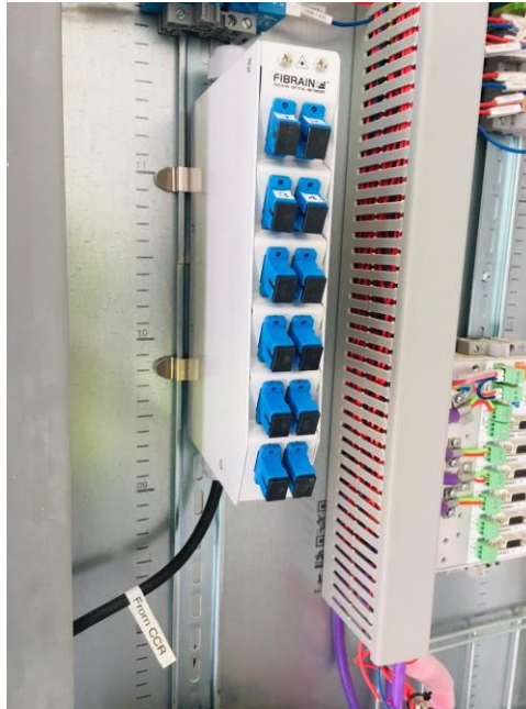
Fig. 4 Fibrain FDM-S-X Din Rail Patch Panel
