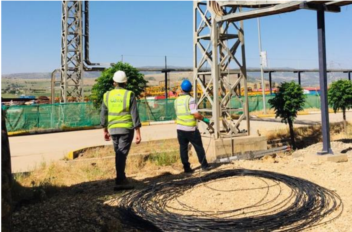
Fig. 2 Roll-out Of Old Cable
